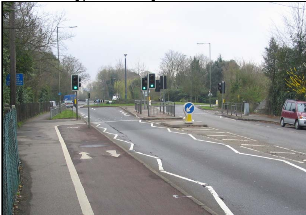
Photo 1 - Existing pelican crossing on Woburn Hill
